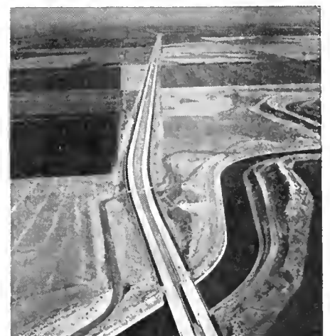
Expressway relocation of US 50 looking easterly toward Tracy, nearing completion. Delta-Mendoto Canal of Central Valleys Project in foreground.
